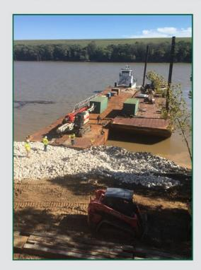
During the demolition phase, the interior of the dock area began it's descent, about 24'. This elevation was the elevation needed for the subsequent phase. It did mean safety precautions, such as constructing safety fencing and establishing measures for preventing fall or fall on hazards.
