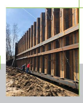
Our next priority was dealing with the drainage and the soil loading. We created a sloped bottom by pumping hundreds of cubic yards of a 150 psi flowable fill with 12" of fall toward the river. This gave us a strong bottom grade to evenly distribute the loads above and ensure water drained towards the river.
