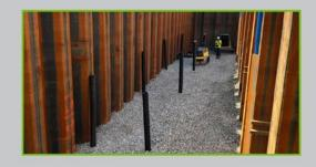
Once the flowable fill cured, we immediately set up a conveyor system to import the free draining, crushed stone. The stone would bed the pipe in place to ensure it was draining through the weepholes in the sheet piles. For maintenance design, piping was installed vertical about every 18' to provide access for flushing of river sediment build up.
