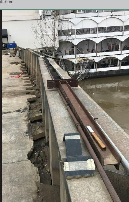
This phase included selective demolition and disposal of the steel and site soils. The site soils were mostly used to balance the erosion that had scoured the area outside of the sheet pile wall. The steel had to be cut out and
