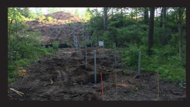
As soon as piering operations were completed on each boardwalk, the general contractor had the framing contractor ready to begin framing operations. Asphalt walkways were then constructed, allowing a smooth transition from asphalt to the pressure treated boardwalk.
