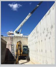
10 piles were beam tested during this project. This included one sacrificial, pre-production pile that was tested to 200% of the design load, or 50-kip Ultimate. This pile test reported 13/16" deflection, which was satisfactory to the engineered specs. Innovative Piering also performed 9 production pile beam tests, which were tested to 100% design load, or 25-kip. All of which passed the requirements with only 3/8" deflection or less.
