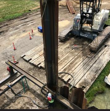
he largest challenge of the project however, was the firm soils that the sheet piles needed to be driven in to. Required driven depths of each sheet was at least 4-6' of embedment. The 'firm' and 'very hard' clays proved to be incredibly challenging to drive the ESZ85 sheets into.
