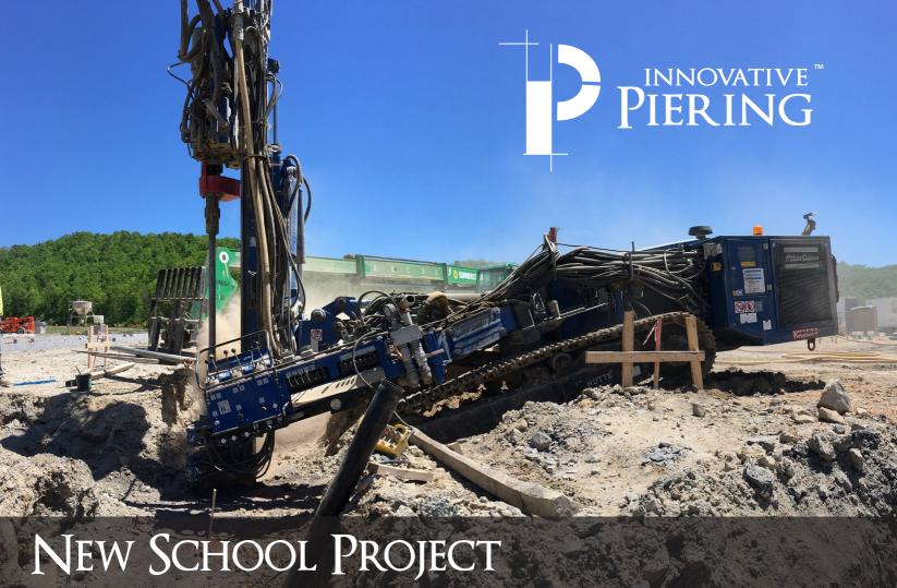
Innovative Piering, LLC was contracted to furnish and install the micropiles required to support grade beams for the new Martin County High School.
