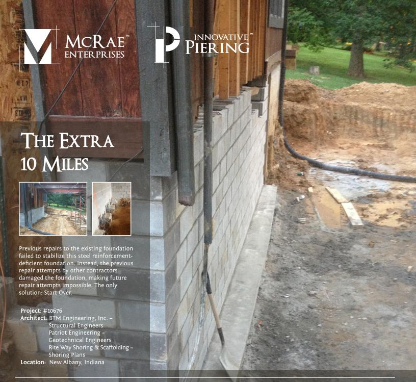
Immediately after evaluating the condition of this home, it was discovered that simple underpinning or repairs wouldn't be a viable option. There were at least three contributing issues. 1) An 8' tall exterior wall was bowed and leaning away from the house with no steel reinforcement in it.
